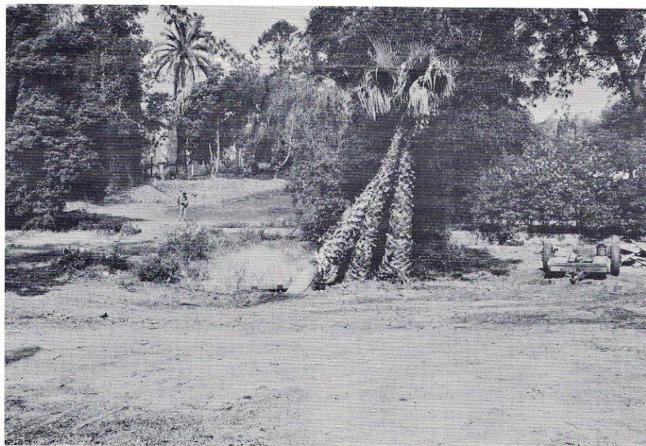
Razed Vernon-Del Mar block awaits transformation into modern physical education plant.
